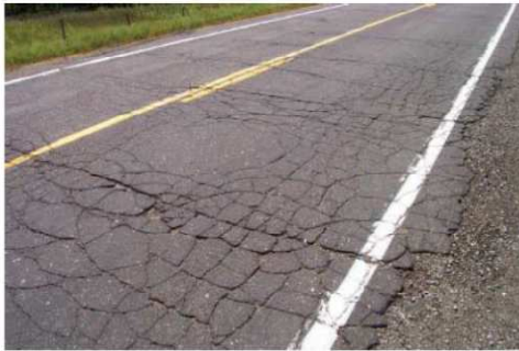
Figure 7.0: Alligator cracking
