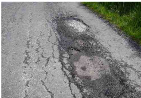
Figure 3.0: Pothole
