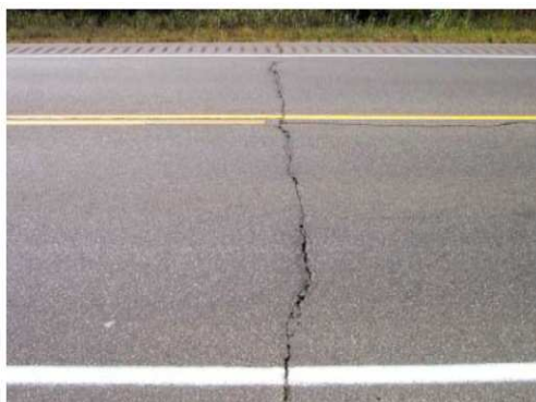
Figure 5.0: Transverse Cracking
